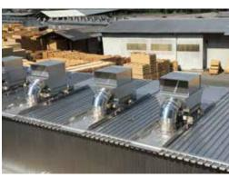
Warm partial airflow that is **not of use** for drying is discharged.
